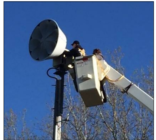
Warning siren repairs are underway!
